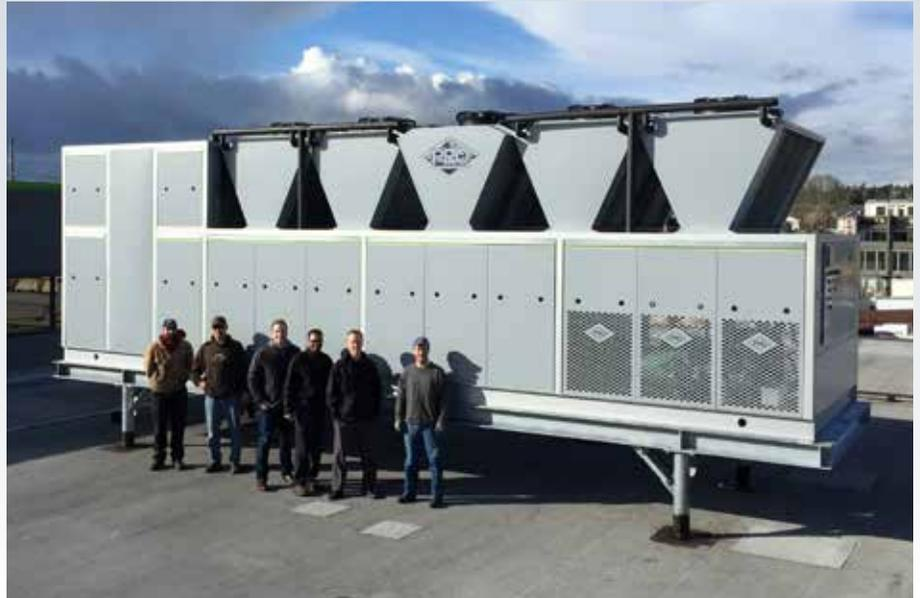
This refrigeration system for process cooling at a brewery uses 5-mm diameter copper tubes in its condenser coils. (Courtesy of PRO Refrigeration, Auburn, Washington)
