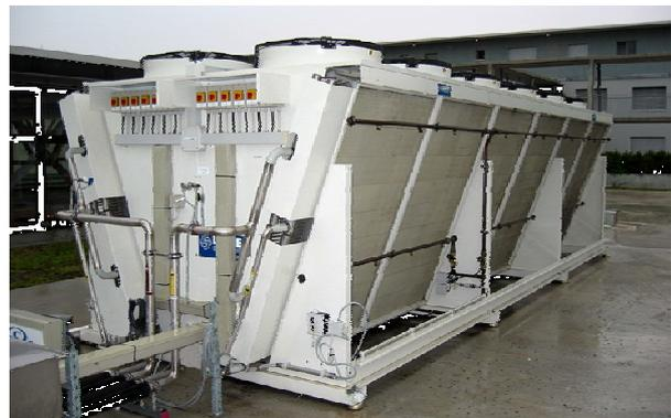
Fig 13 –  $CO_2$  gas cooler with spray (summer capacity = 500kW)
